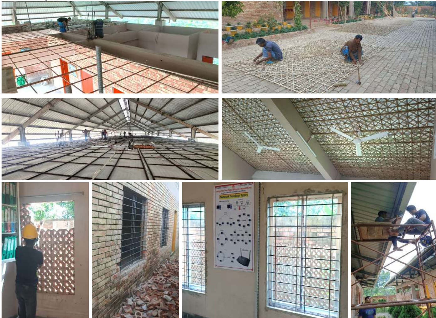
Campus Renovation Work
