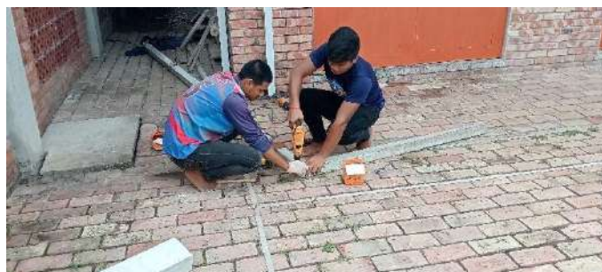
Students Repairing Drain Line
